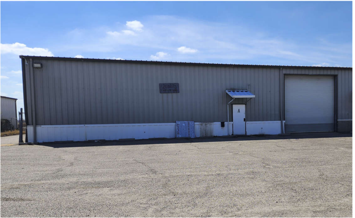
FIGURE 5 View of Building East Elevation
