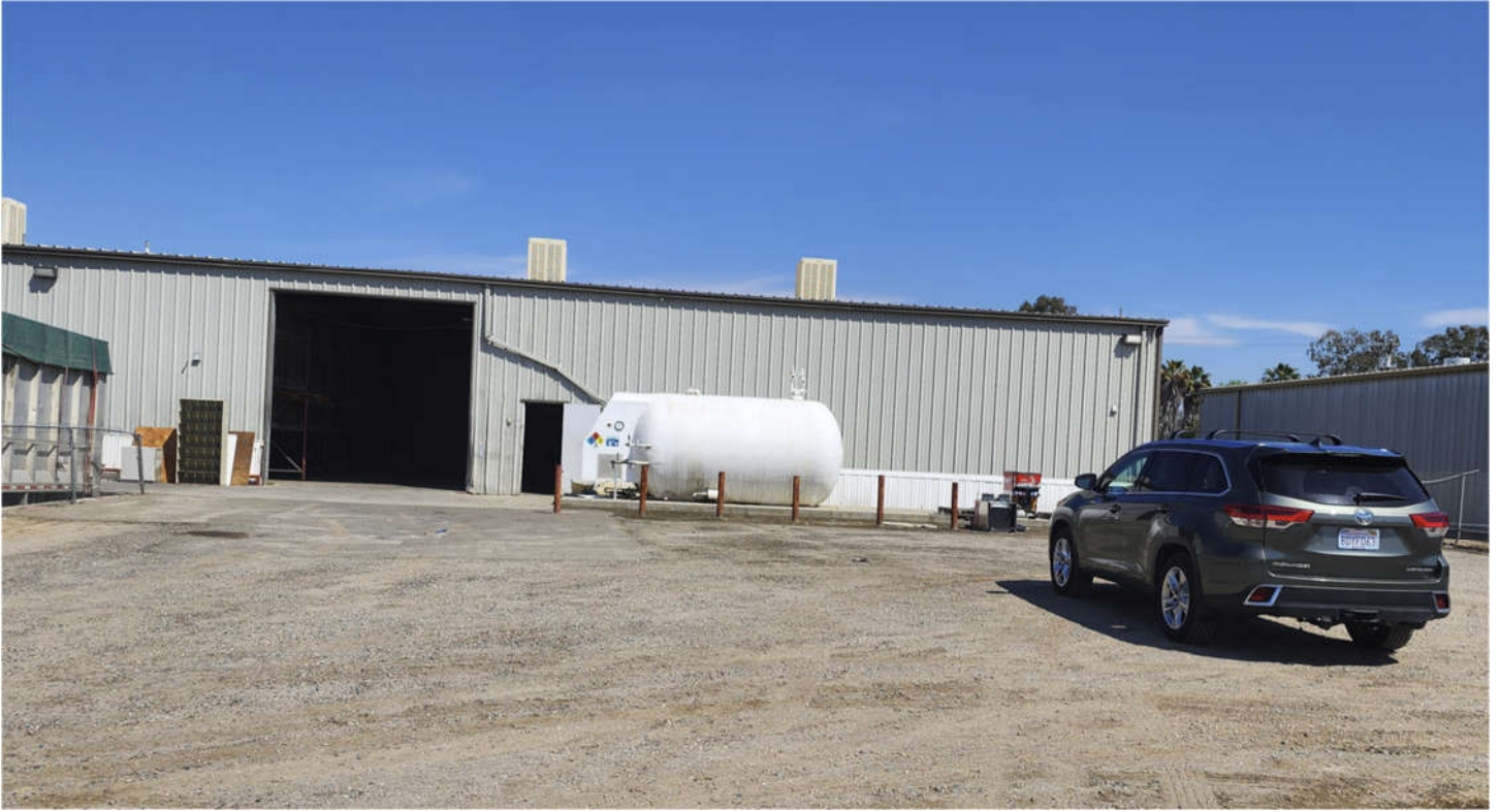
FIGURE 7 View of Building West Elevation (Tank is not part of this application and will be removed)
