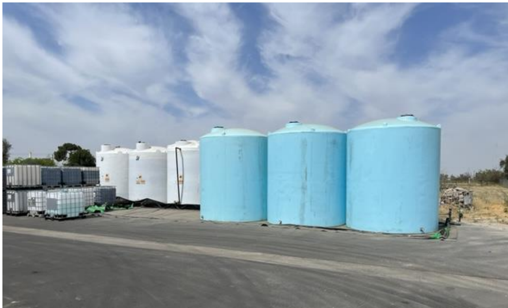
Outside storage tanks and totes. Tyvek containment in place beneath tanks.
