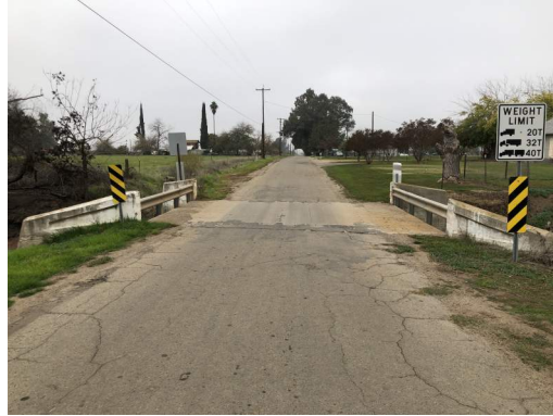
Figure 2 View of the existing bridge facing west.
