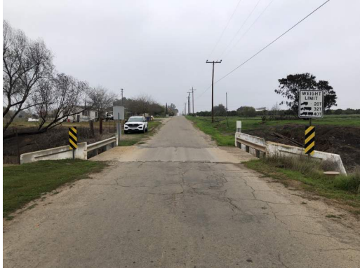
Figure 1 View of the existing bridge facing east.
