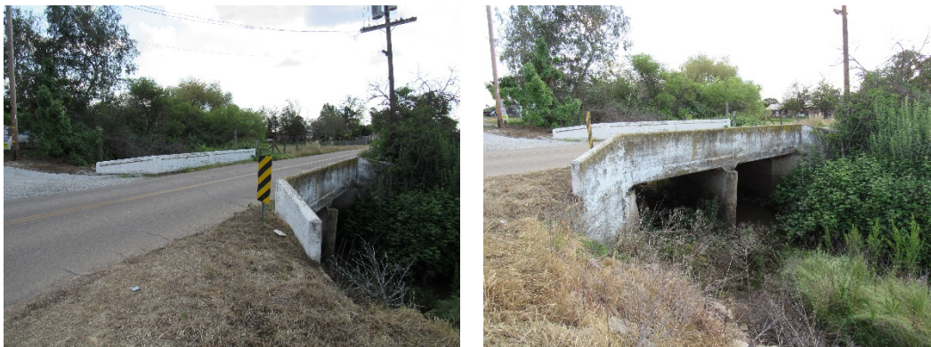
Figure 1.3: Existing Parlier Avenue Structure
