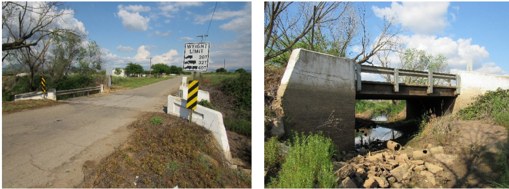
Figure 1.2: Existing Lincoln Avenue Structure
