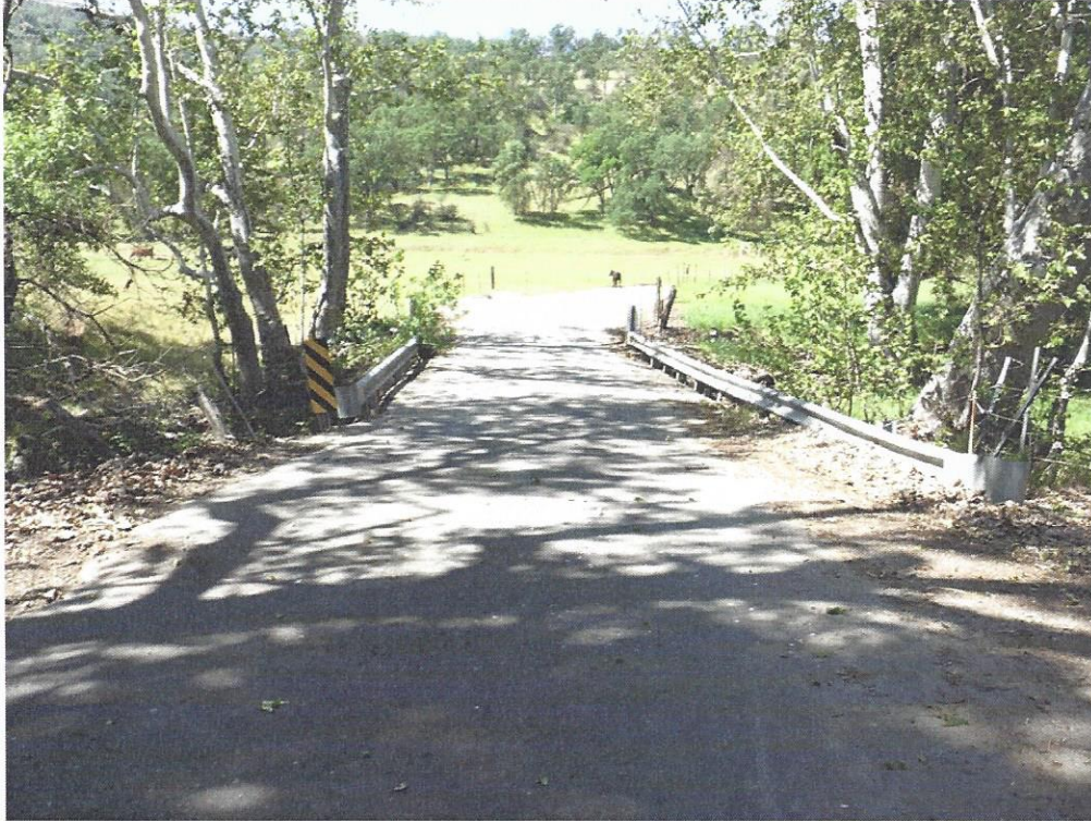
Photo No. 1 Looking south.
