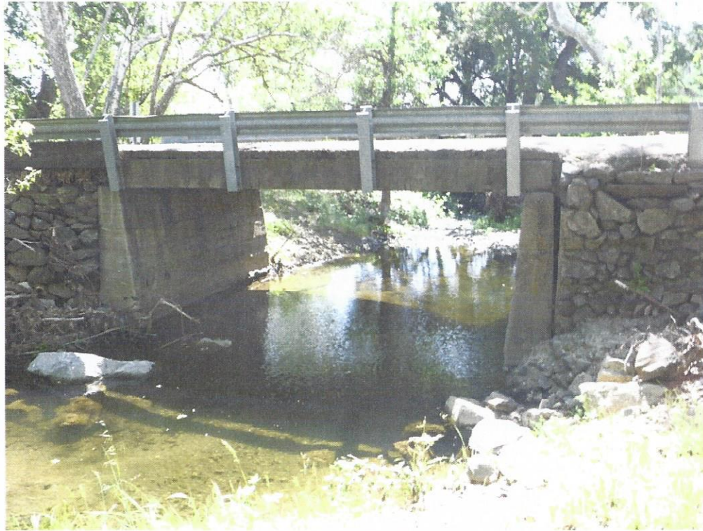
Photo No. 2 Looking east.
