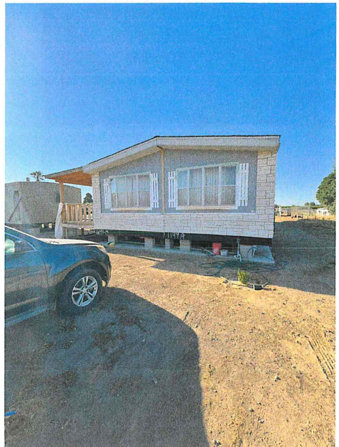
SOUTHERN SIDE OF MOBILE UNIT FACING NORTH
