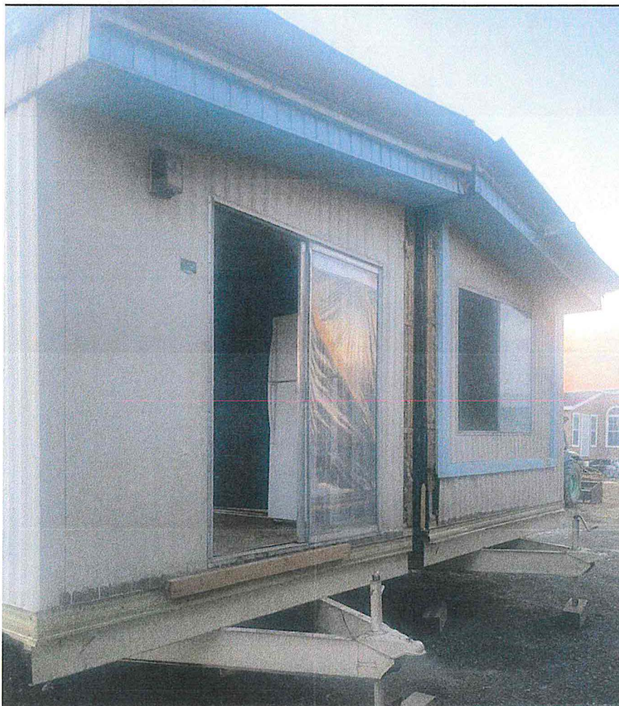
BACK END OF MOBILE HOME, WILL BE FACING EAST WITHIN PROPERTY.
