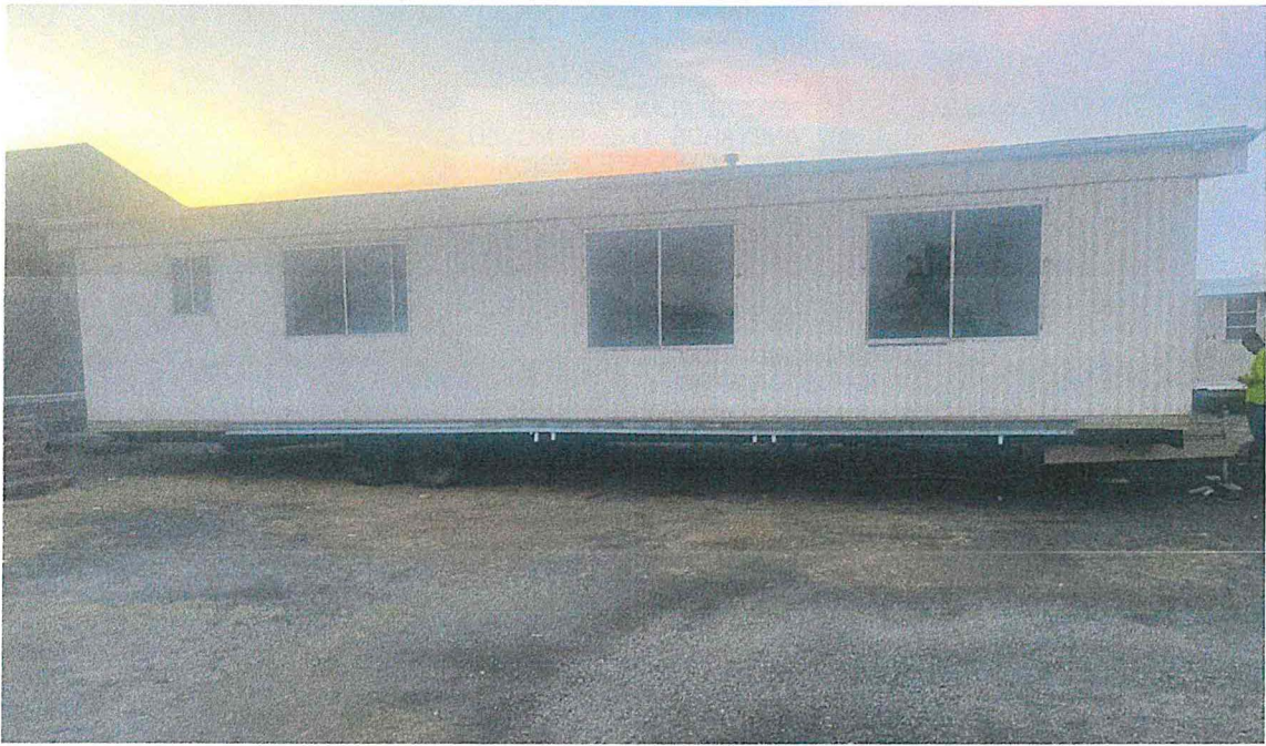
SIDEVIEW OF MOBILE HOME FACING SOUTH ONCE PLACED WITHIN PROPERTY.
