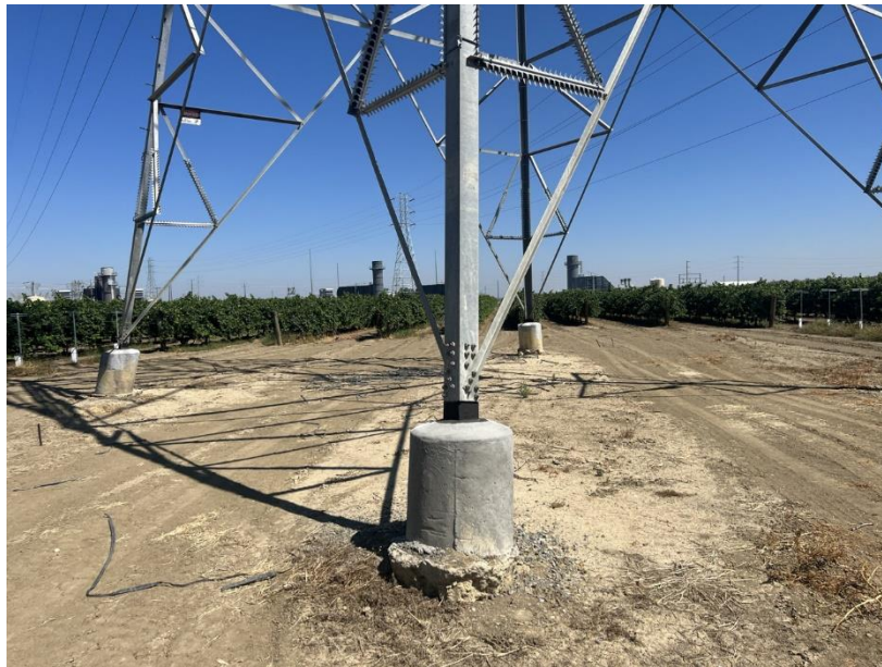
Photo 1 The base of resource P-10-006614 surrounded by grapevines, Facing North.
