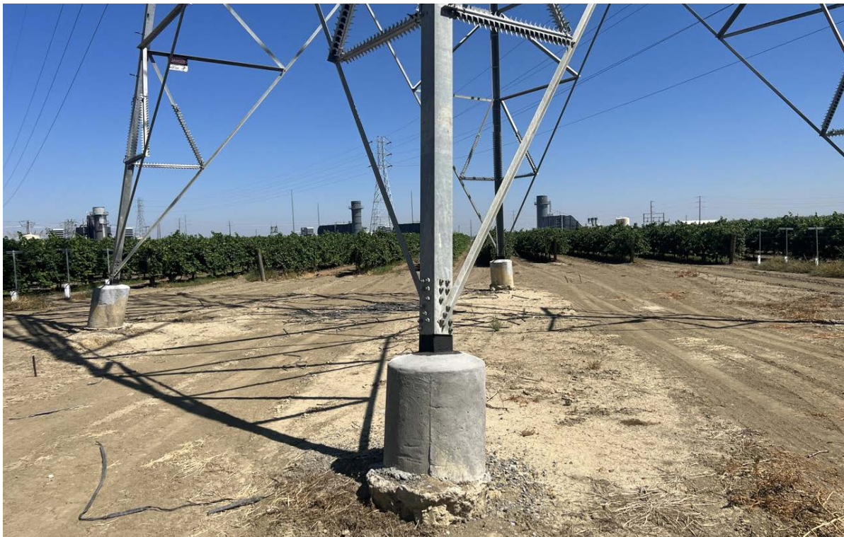
Figure 4 P-10-006614. Panoche Kearney 230 kV Transmission Line, View North
