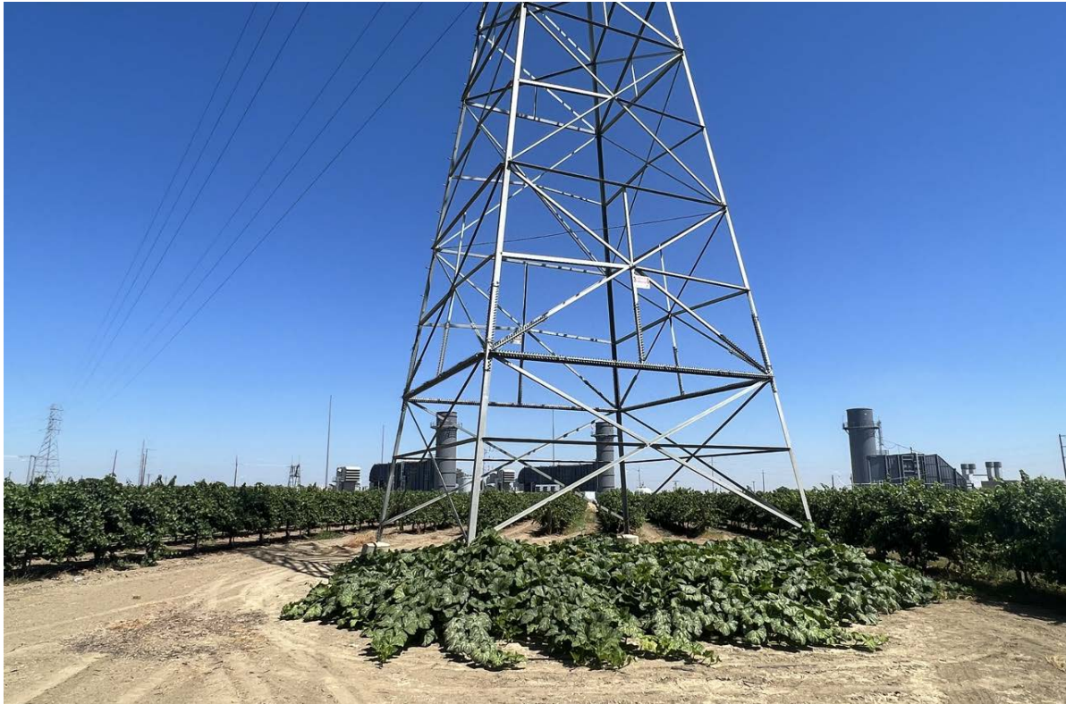
Figure 3 P-10-006612. Schindler-Panoche 115 kV Power Line, View North
