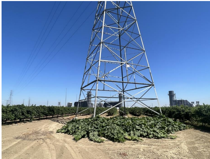
Photo 1 The base of resource P-10-006612 surrounded by grapevines, Facing North.
