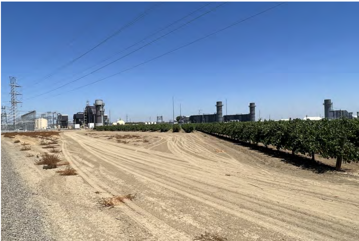
Photograph 2. South Central Boundary of the Project Area looking towards the Panoche and Midway Peaker Plants, View Northwest.
