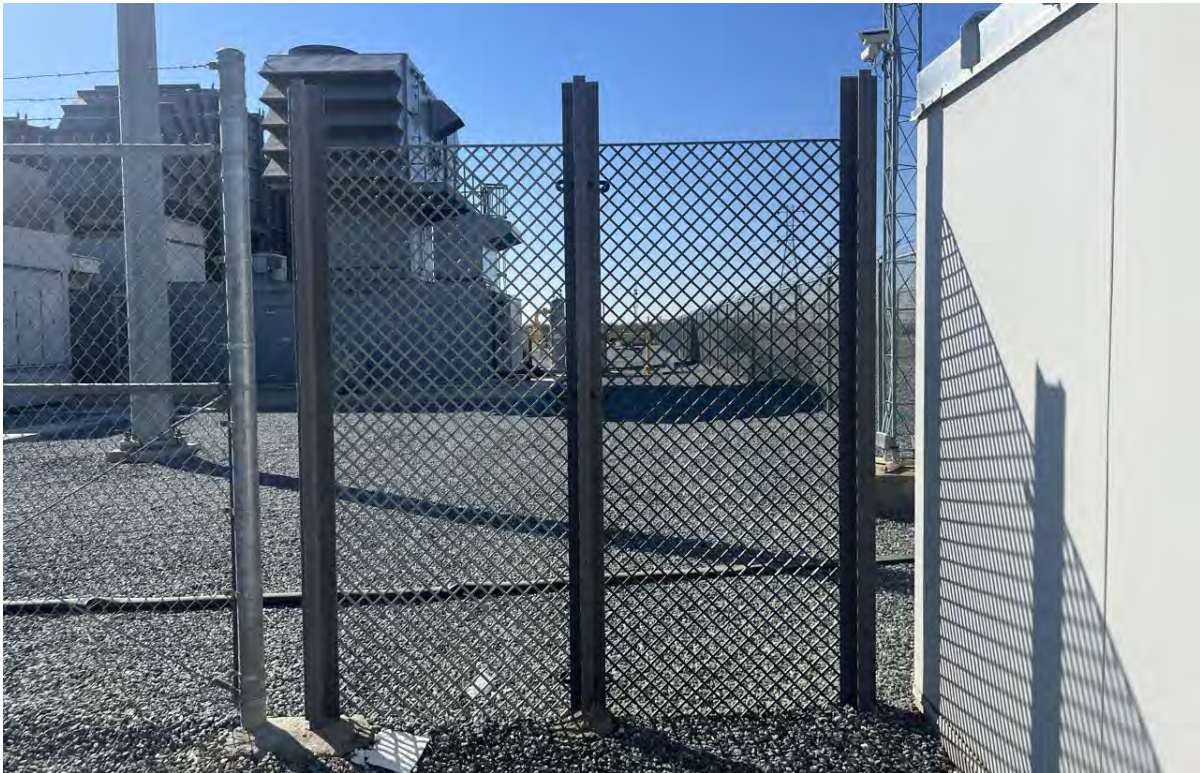
Photograph 4. Overview of Current Midway Peaker Plant Facility, View South.
