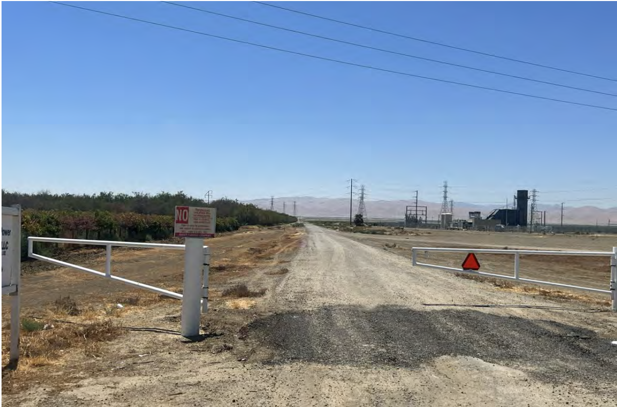
Photograph 3. Overview of Northeastern Boundary of the Project and access road, View South.
