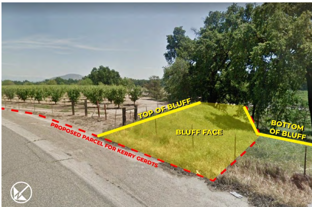
Street View Illustrating Bluff Slope
