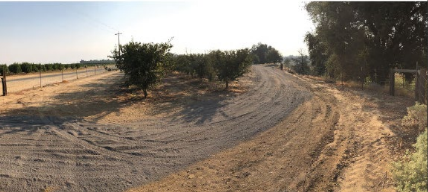
Existing Farm Service Road
