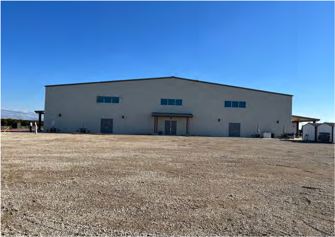
Site Photo View B - Facing East toward Existing Gym
