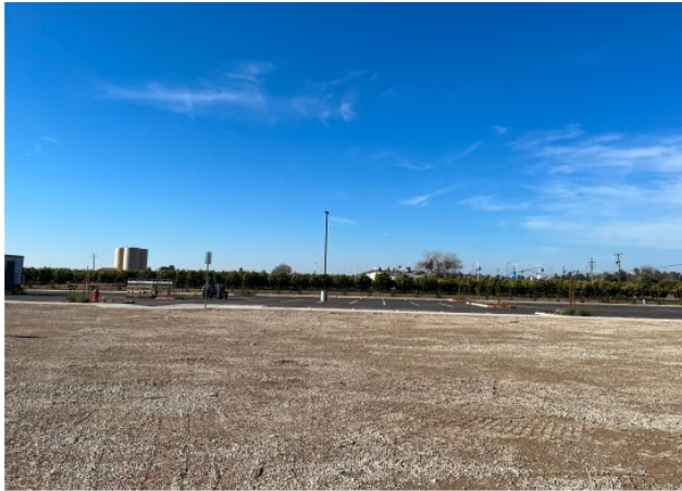
Site Photo View D - Facing West towards parking and Academy ave beyond
