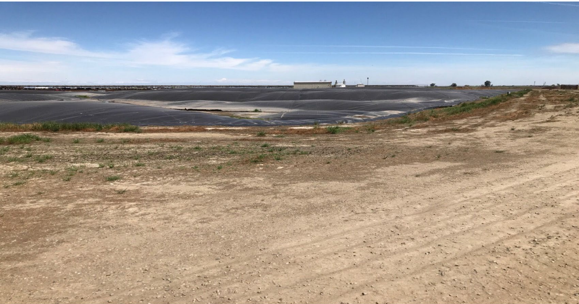
Covered lagoon digester on Open Sky Dairy, facing northeast.
