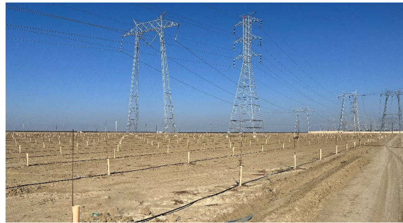
Photograph 2. View of the electrical transmission lines along the eastern subject property boundary.
