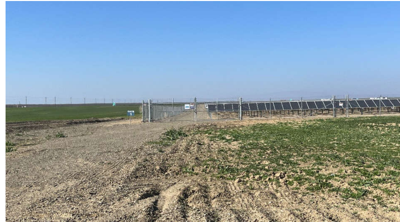
Photograph 16. View of the western adjacent solar array, facing west.
