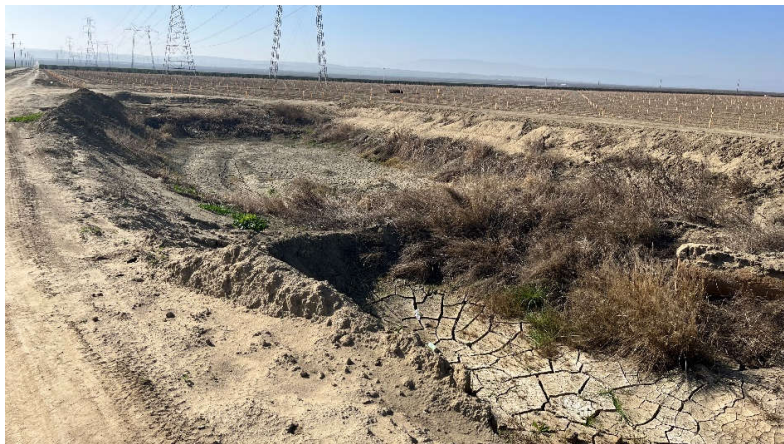
Photograph 3. View of the drainage ditch in the northeastern corner of the subject property.
