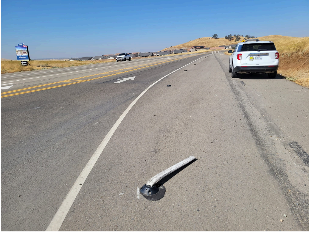
Figure 1: Facing west on Millerton Road from Winchell Cove Road. Roadside pylons have been flattened or broken off completely by vehicles attempting to merge.
