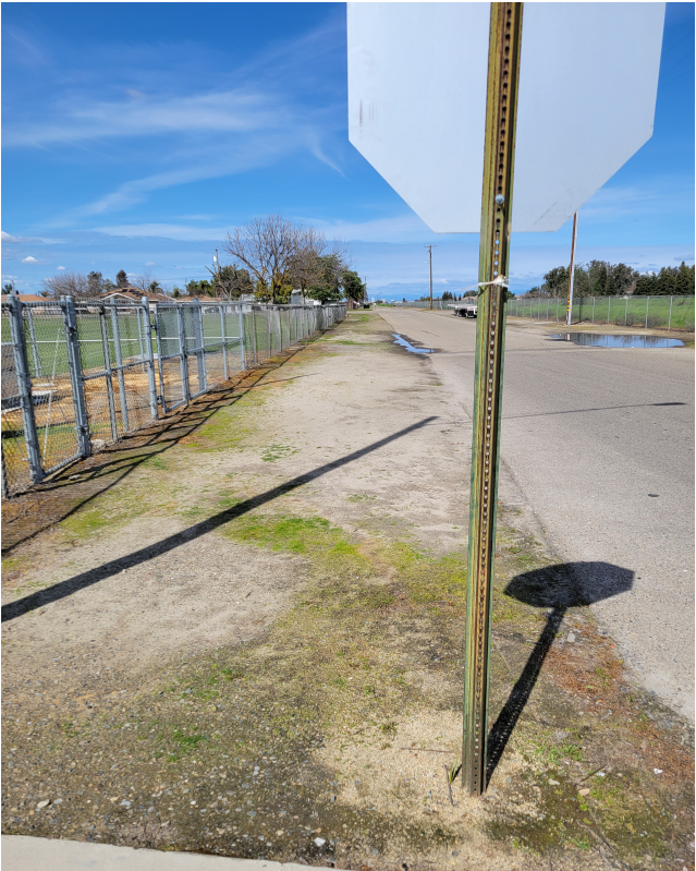
Figure 6: West side of Lily Ave facing north at elementary school.
