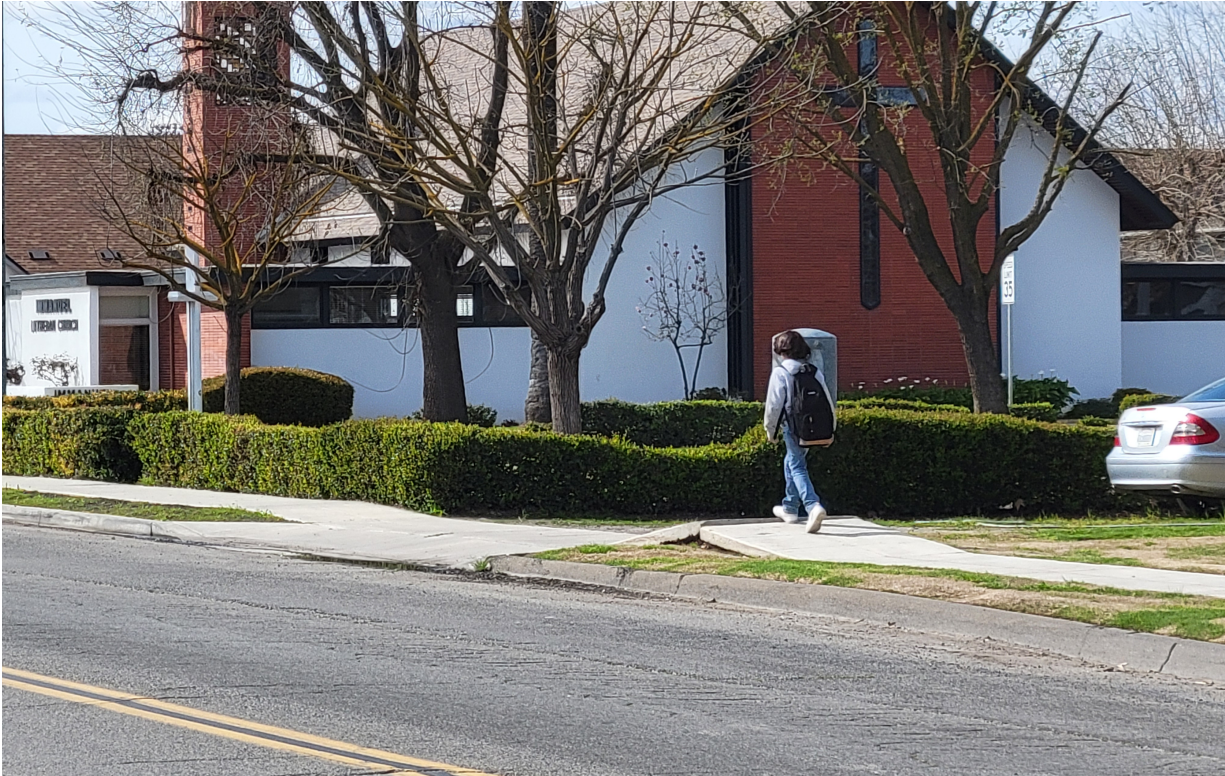
Figure 1: Student walking on buckled sidewalk on north side of Lincoln Ave near elementary school.
