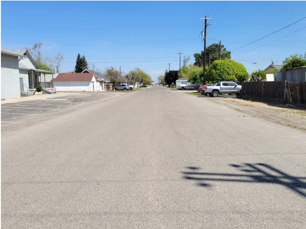
Figure 12: Superior Ave facing NE from Raider Ave (fairgrounds).
